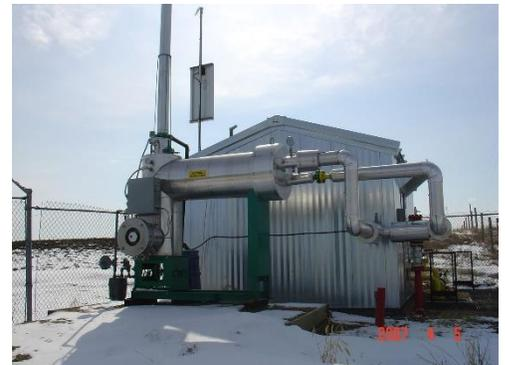
Figure 15 - Natural Gas Fired Heater
